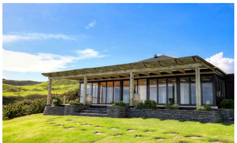
Main Cliff Top Venue Exterior
